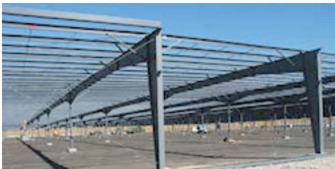
Steel for covered parking structure made from 35% recycled cars.
